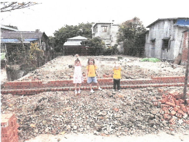
The completed brick foundation for the walls and completed drainage ditch.
