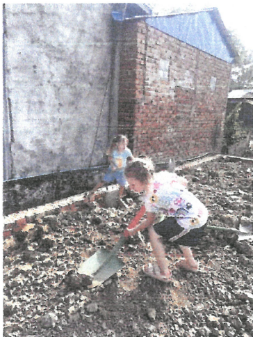
The completed brick foundation for the walls and completed drainage ditch.
